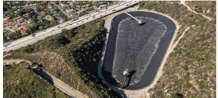
The floating cover on the Eagle Rock Reservoir provides added protection to L.A.'s drinking water.
